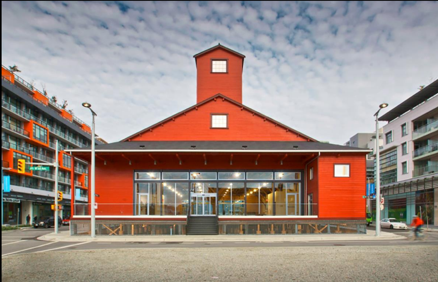
Front elevation with new large windows for receiving maximum daylight, credit: Acton Ostry Architects
