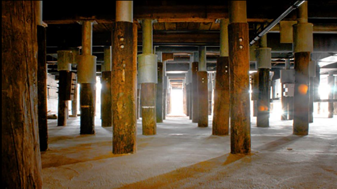
Building raised with steel pile extensions, credit: Acton Ostry Architects
