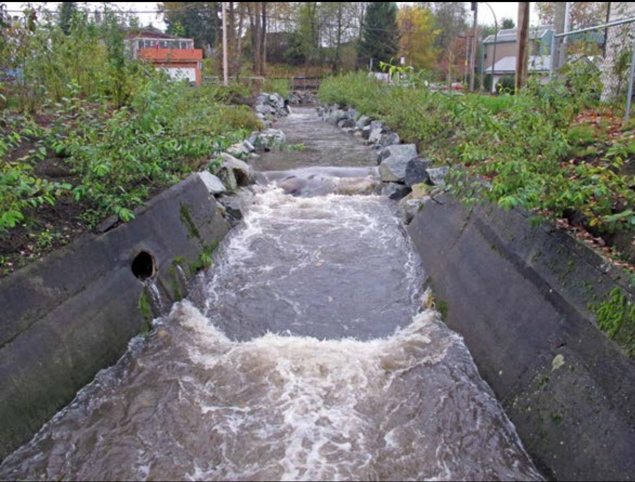
Above: A section of Still Creek next to the Grandview Highway demonstrating the change between the original concrete banks and new naturalized banks. Credit to Bob Kronbauer, 2012
