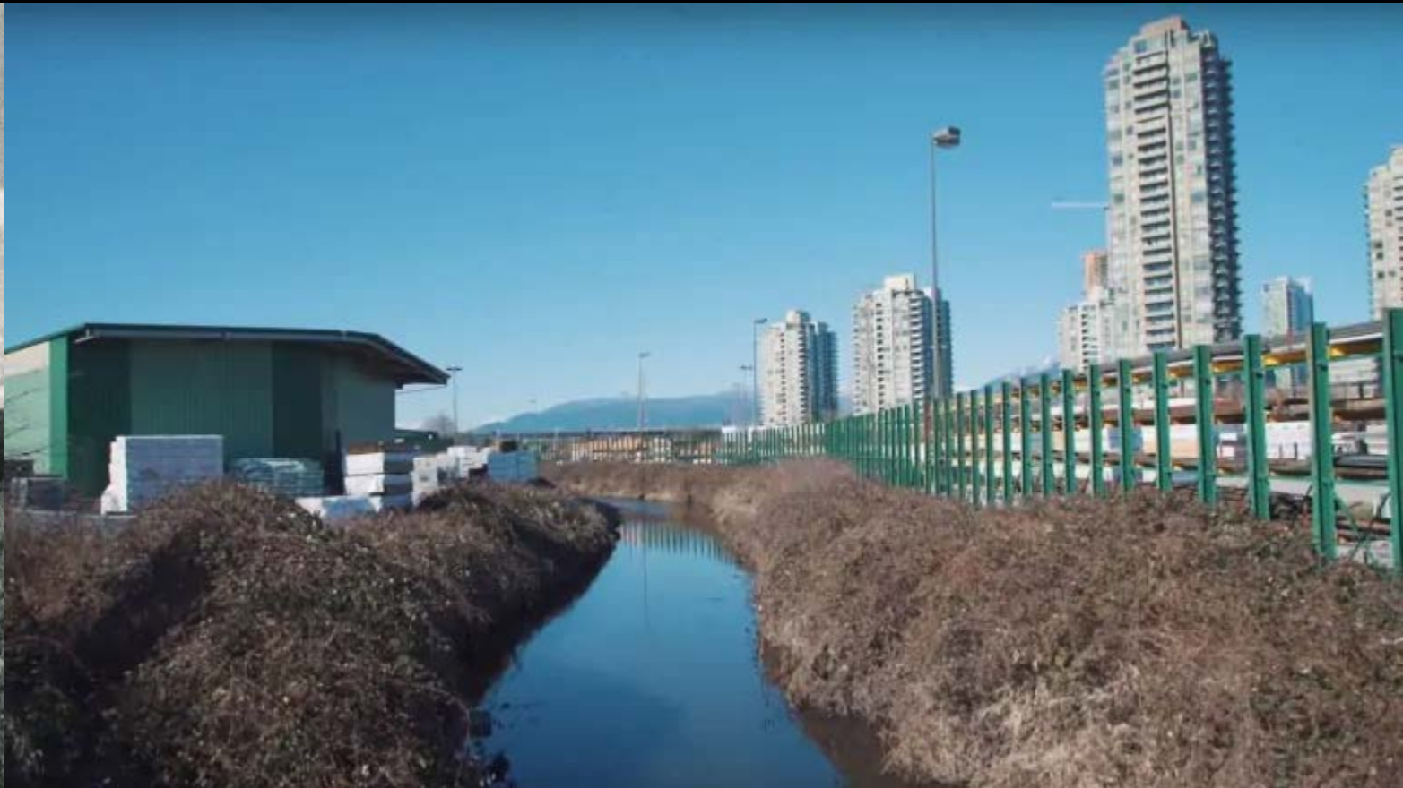
An open section of Still Creek before restoration, note the engineered Banks and riparian zone completely overgrown with a single invasive Species. Credit to Uytae Lee and the CBC, 2019.
